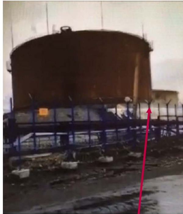
The dynamic force of the diesel release resulted in the overtopping of the bund wall
