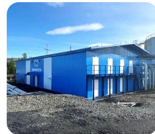
Modular treatment facilities for suspended solids, discharge point 170, Oktyabrsky mine
