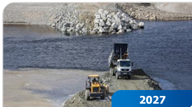
Construction of a new water intake on the Norilskaya river
